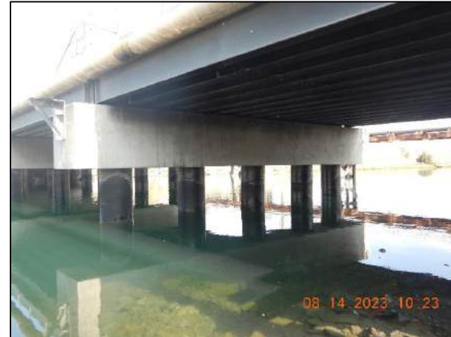
Photo No. Note: Typical Bent 2
