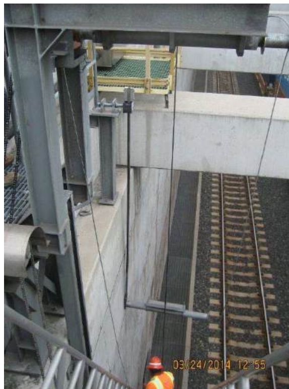
Lower End Counterweight – Down Position
