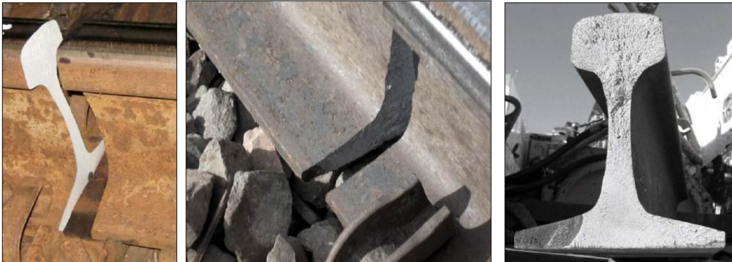
Broken Base – Transverse Photo Examples of Broken Base - Transverse
