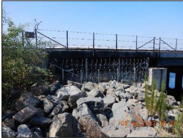
Photo No. Note: Span #1 and #6 not accessible 1
