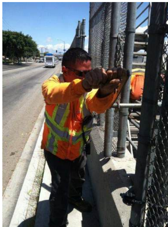
Cranking from Street Level
