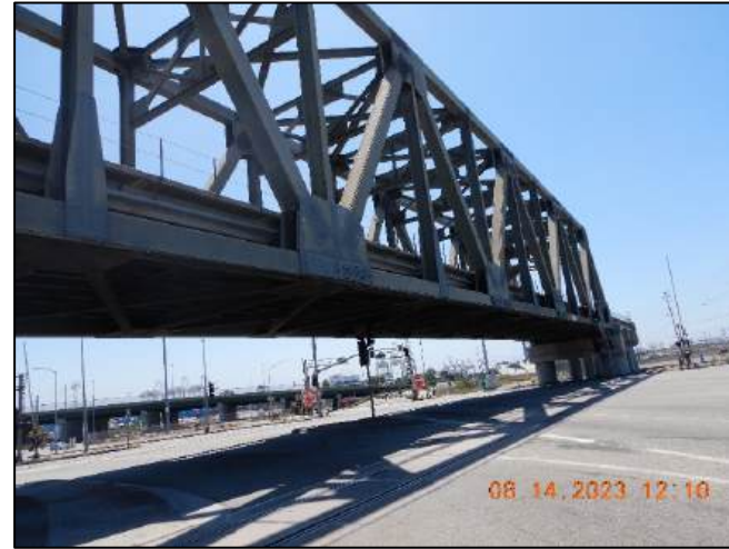
Photo No. Note: Span 3 - Second through truss span over road. 2
