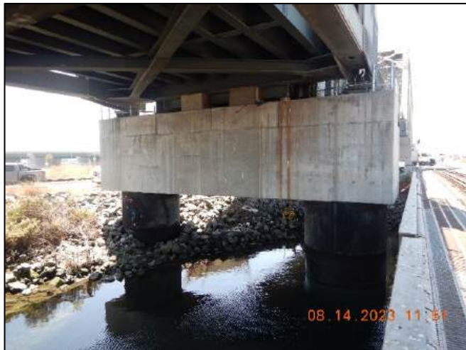
Photo No. Note: Underwater column repairs around column wraps 3
