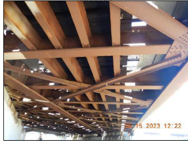
Photo No. Note: Floor system and bottom lateral bracing. 2
