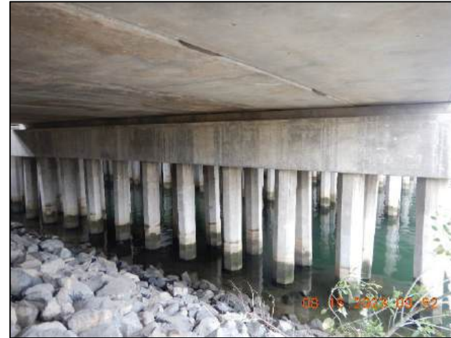
Photo No. Note: Typical concrete end span. 2
