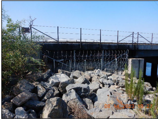
Photo No. Note: Span #1 and #6 not accessible 1
