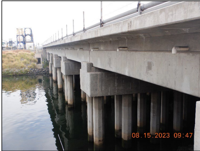
Photo No. Note: All concrete bents composed of columns and caps. 1
