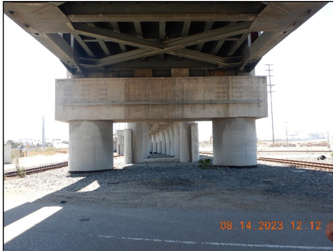
Photo No. Note: Typical two column concrete bents. 5
