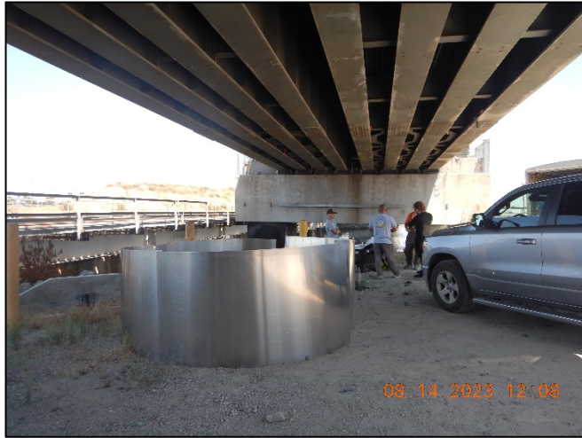
Photo No. Note: Underwater column repairs around column wraps 1
