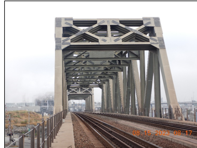
Photo No. Note: Typical Truss bays, in good condition. 6
