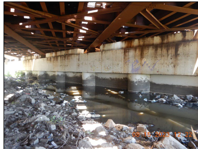
Photo No. Note: Typical substructure. 4
