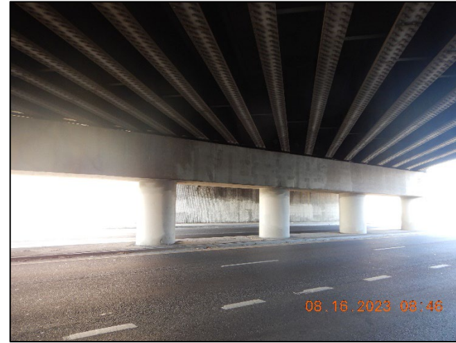
Photo No. Note: Cap at concrete bent. 6
