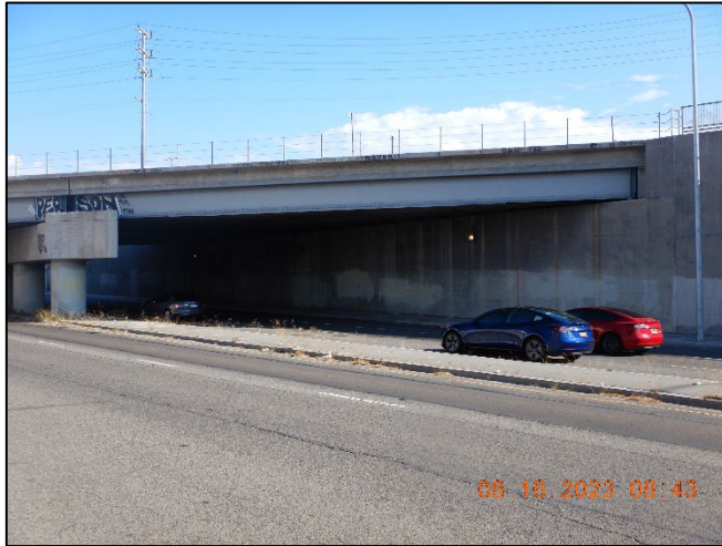
Photo No. Note: Right side of bridge, missing overhead vertical clearance sign. 1
