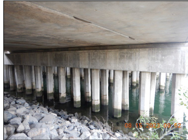
Photo No. Note: Typical concrete end span. 2
