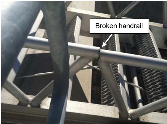
Ladder #2 (Repair later completed)
